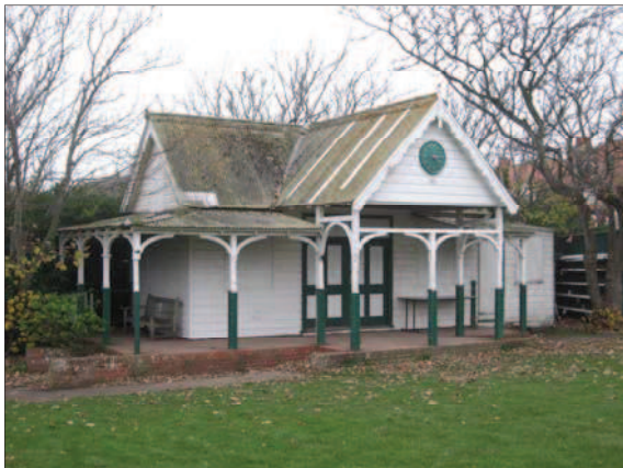
Curtilage listed sports pavilion
