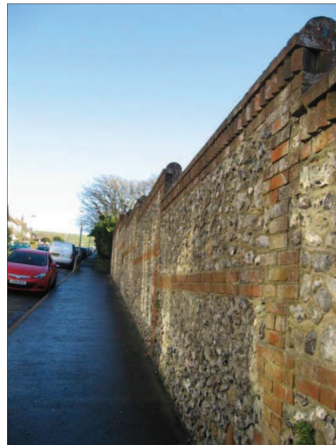
The flint and brick wall along Steyning Road
