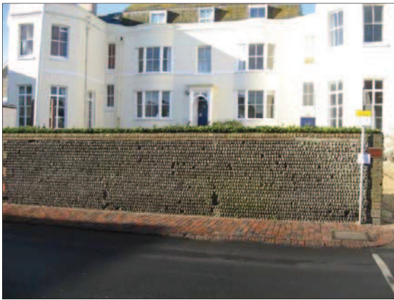
Grade II listed flint wall on western boundary
