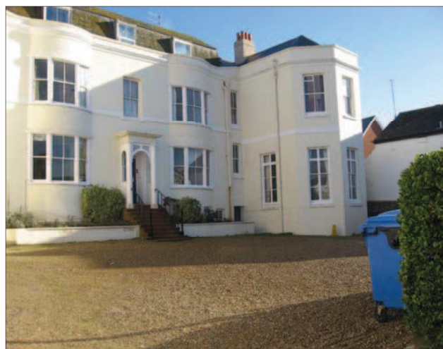
Small car parking area
